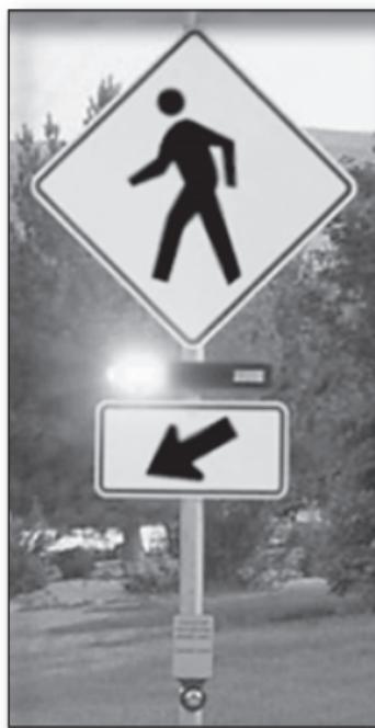
Rapid Flash Beacons (RFB) combined with pedestrian crossing signs are installed at specific crossings to alert drivers to the presence of pedestrians. When pedestrians activate the push button system, yellow LED lights begin a random flashing sequence to alert drivers to the presence of pedestrians at the crossing. When not in use, the RFB will remain dark.
